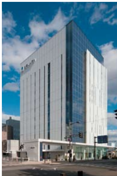
KITAMI SHINKIN BANK, Head Office
